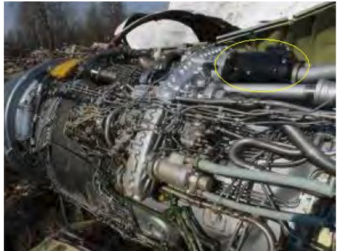
Fig. 14. Generator ГТ40ПЧ6 on Nr 1 (left) Д-30KY turbopan engine. Photo taken between 11 and 13 April 2010 on the crash site [4].
